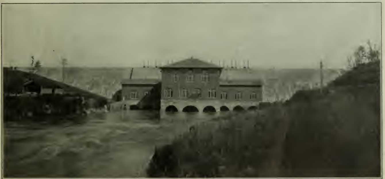
FIG. 1. VIEW OF GREAT FALLS STATION AND DAM FROM THE TAIL STREAM
